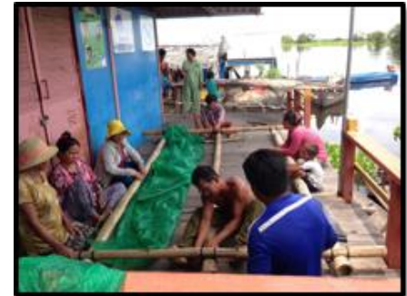
Constructing floating gardens on Tonle Sap Lake
